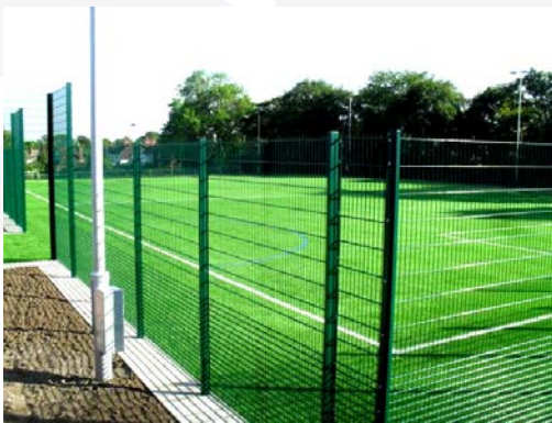
Example of resistance mesh panel fencing Floodlights
