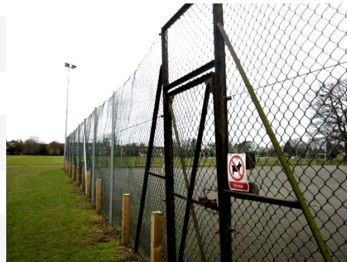
Perimeter ball-stop fencing
